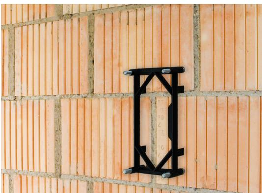
Insert the threaded rods and precisely align them by pushing in the respective setting jig.
