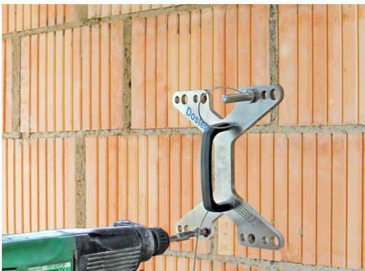
For the drilling jig for SLK®-ALU-TR / -TQ, insert a positioning bolt into the corresponding hole.
