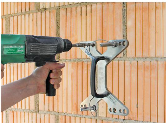
For the drilling jig for SLK®-ALU-TR / -TQ, insert a second positioning bolt into the corresponding hole.
