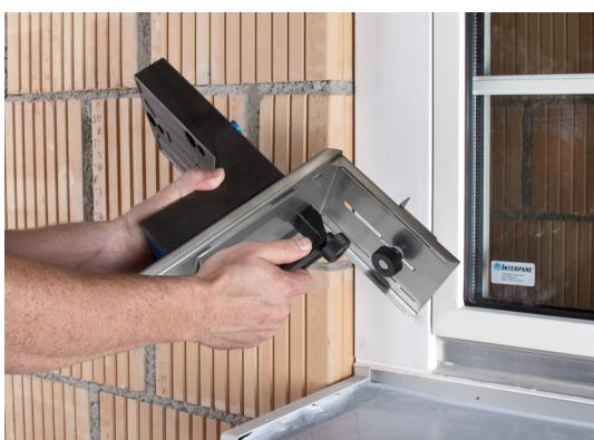
Slide the jig up to the K1-PE, K1-PU bracket support element or the supporting bracket TRA-WIK®-PU.
