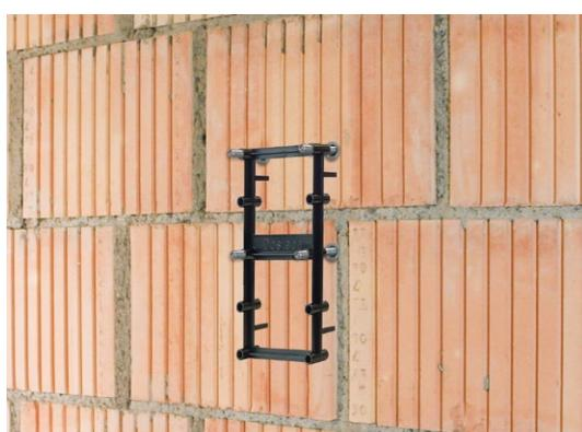
Position the threaded rods and align them exactly by inserting the respective setting jig.
