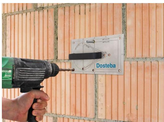
With the drilling jig for UMP®, TRA-WIK® and TWL®, insert a threaded rod into the corresponding hole.
