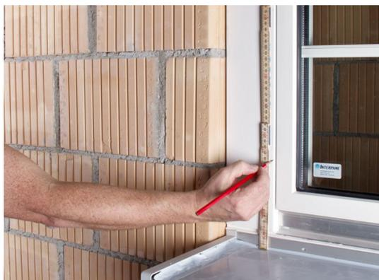
It is advisable to offset the K1-PE bracket support elements and supporting bracket TRA-WIK®-PU before gluing the insulation panels.
