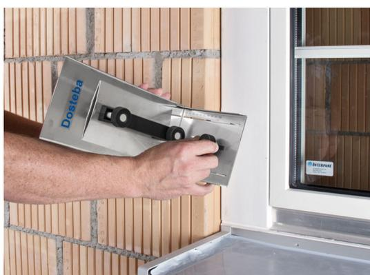
Set the gauge to the desired visual frame dimensions.
