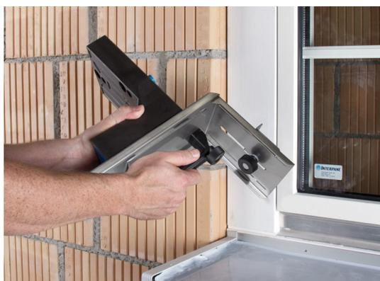
Slide the gauge up to the K1-PE bracket support element or the supporting bracket TRA-WIK®-PU.
