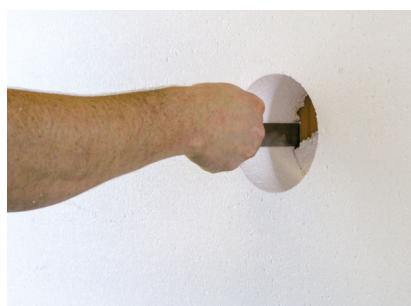
Scratch out residual thickness with suitable tool and remove any milled dust.
